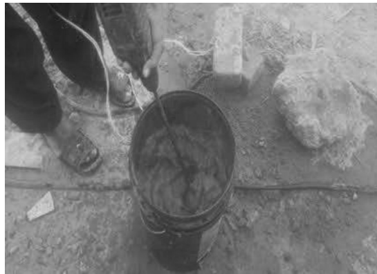
Fig. 2 Mixing of PPPMS slurry with water
