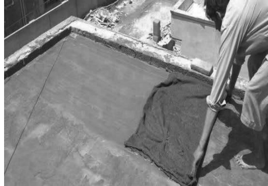
Fig. 6 Grouting of joints
