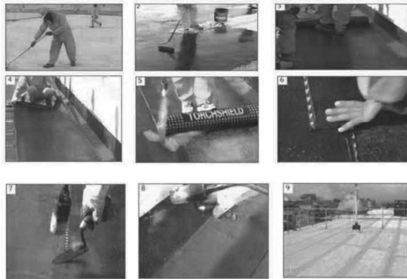
Fig. 1 Waterproofing for roofs with bitumen felt
