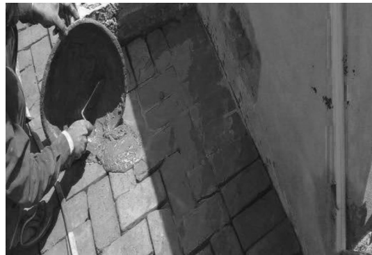
Fig. 7 Smoothing of cement grouting
